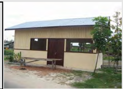
Fasilitas Eco Center RT 16 KAP
